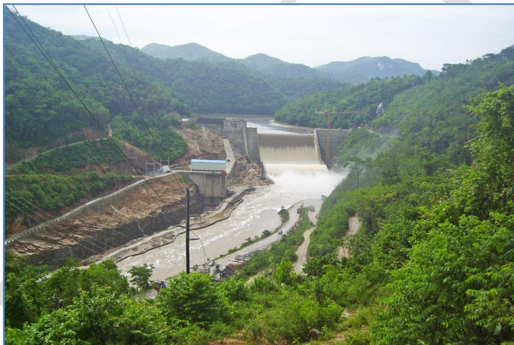
Figure 3.1.10: The Chalillo Hydro Plant is part of a 50 MW cascading scheme on the Macal River in Belize
